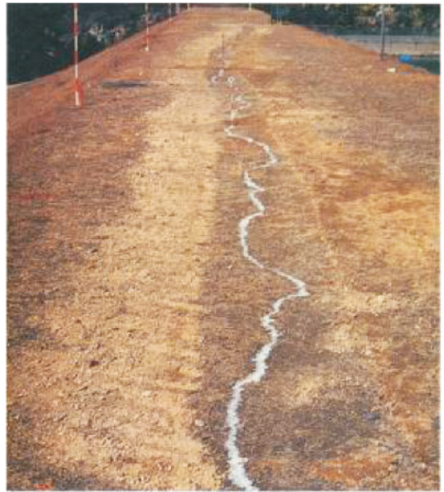
Figure 6. Open crack in direction parallel to dam axis (Hyogo Pref. 1996).
