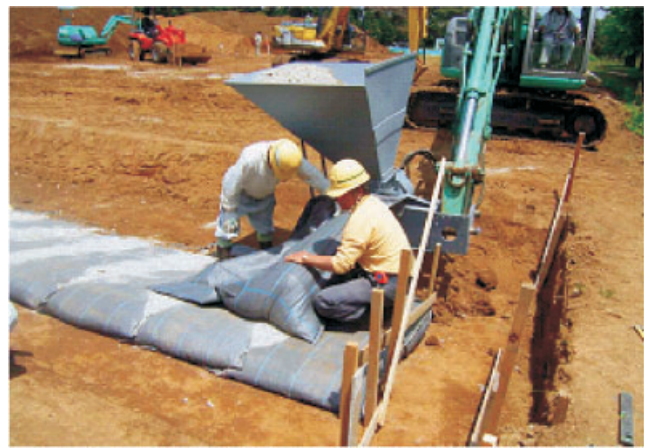
Figure 45. Typical screw extruder for filling soil bags (after Mohri et al. 2007)
