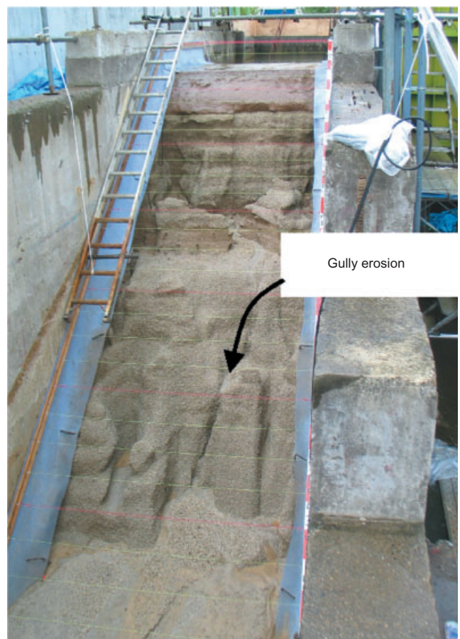
Figure 24. Erosion trace on unreinforced soil slope after 5 min at q = 0.050 \text{ m}^3/\text{s}/\text{m}
