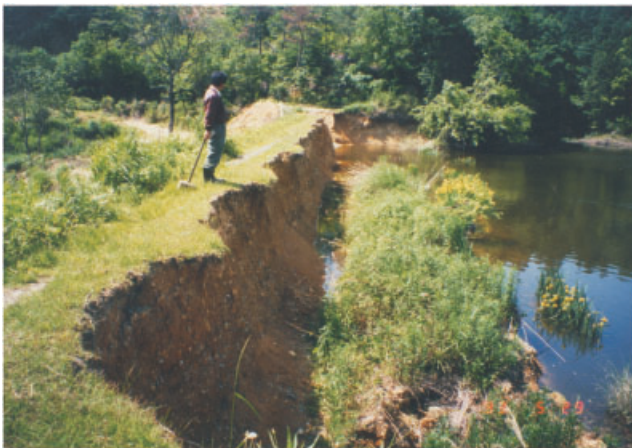
Figure 5. Upstream slope sliding by seismic loading (Hyogo Pref. 1996)
