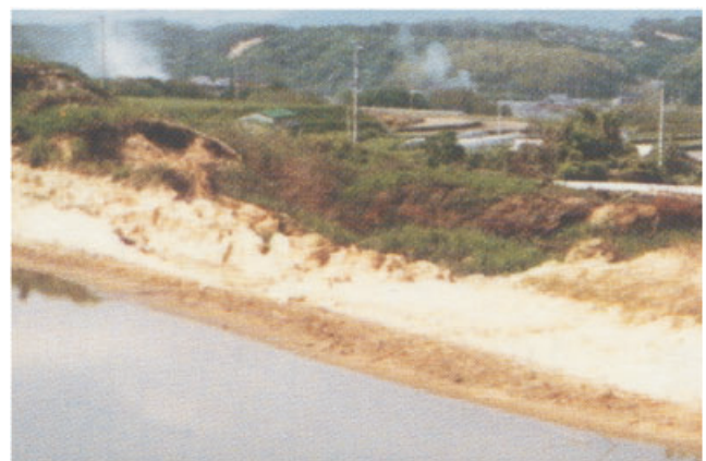
Figure 4. Total failure and large settlement caused by Kobe earthquake, due to liquefaction (Hyogo Pref. 1996)
