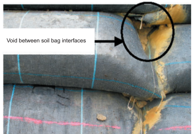
Figure 20. Evidence of sucked backfill material in cell zone behind stacked soil bags
